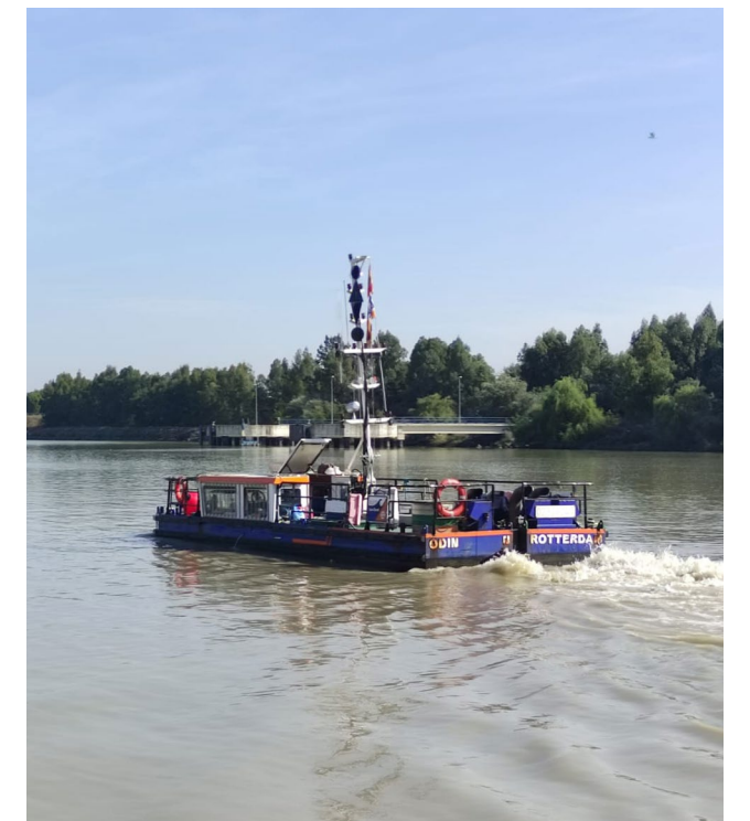
Piloto Water Injection Dredging, WID.
